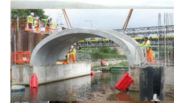
Elland Bridge Repair
